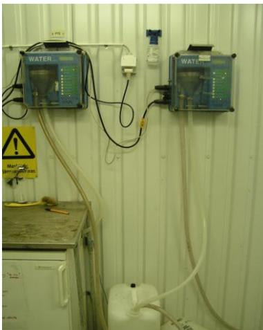
*Figur 2 Sampling point effluent wastewater*
