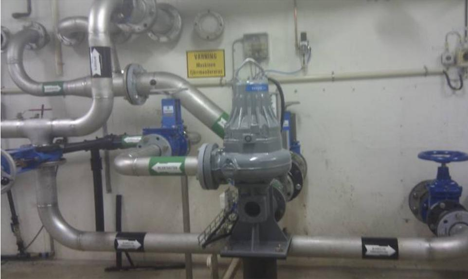
**Figure 2.** Reject water pump. Dosing today the pre sedimentation with reject water.
