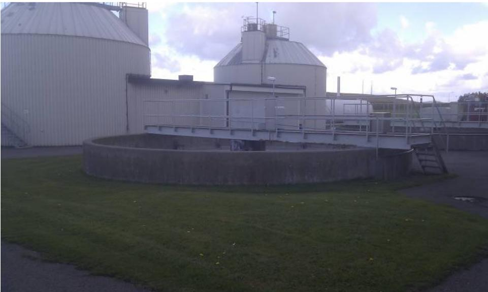
**Figure 1.** Reject water tank and thickener. In the background are the plant two reactors and the torch.
